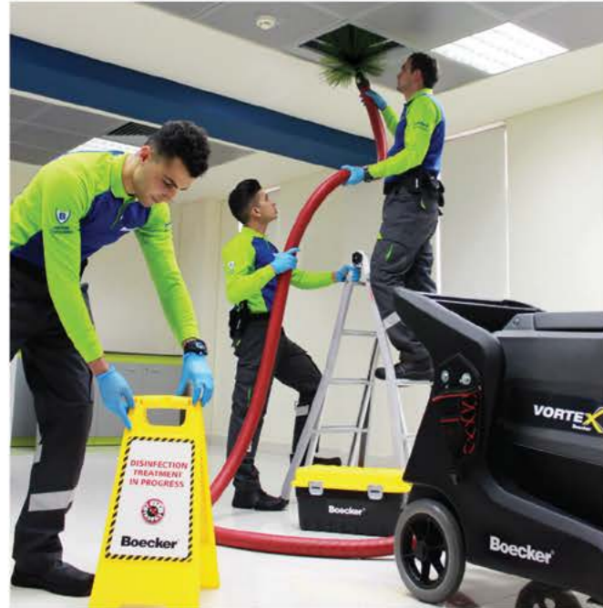
Cleaning air ducts using the latest technology with live monitoring.
