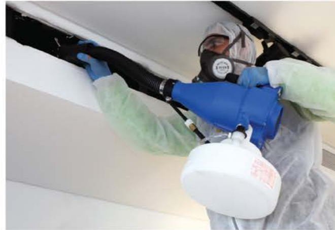
Disinfecting air ducts with safe and certified products.
